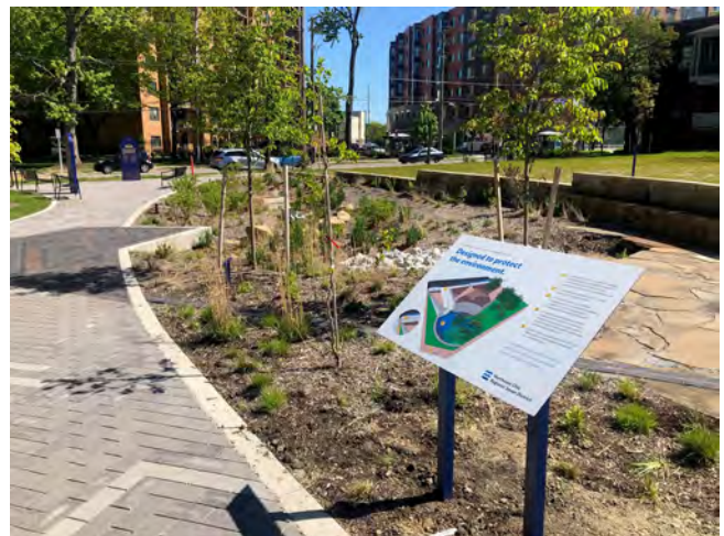
Bioretention and porous pavement walkway at Cozad-Bates House in University Circle. Paid for with grant funding from the Northeast Ohio Regional Sewer District.
