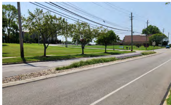
Memphis Avenue after installation of road diet and beautification project (City of Brooklyn.)
