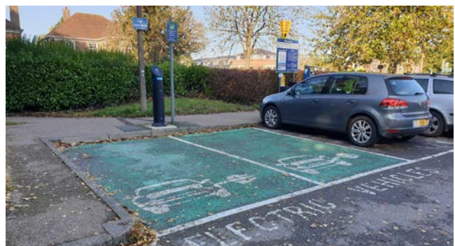
EV Charging Station at a parking lot. Source: OrangeStarling1997 https://commons.wikimedia.org/wiki/File:Chequer_Mead_Electric_Vehicle_Charging_Station.jpg File:Chequer_Mead_Electric_Vehicle_Charging_Station.jpg
