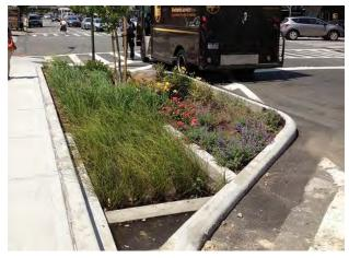
This curb bumpout shows an example of green infrastructure, in which stormwater is directed to natural areas rather than storm sewers.
