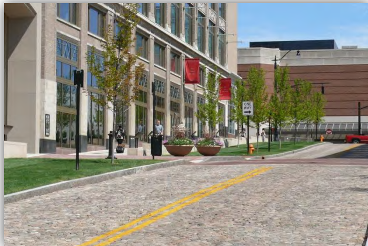
Figure 32: Permeable Pavers Columbus, Ohio
