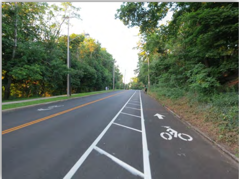
Figure 29: Buffered Bike Lane, Edgehill Road, Collaboration of Cleveland and Cleveland Heights, Ohio
