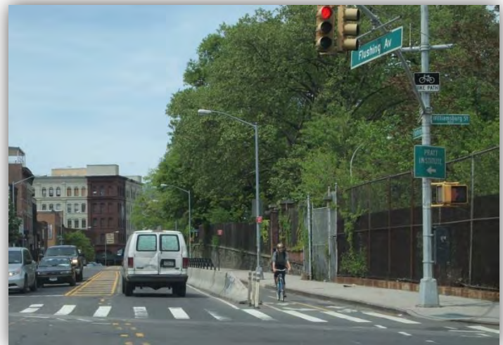
Figure 27: Protected Contra-Flow Bike Lane in N.Y.C.
