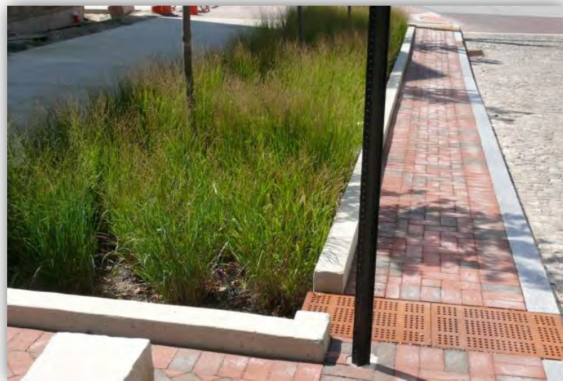
Figure 33: Biofilter, Columbus, Ohio
